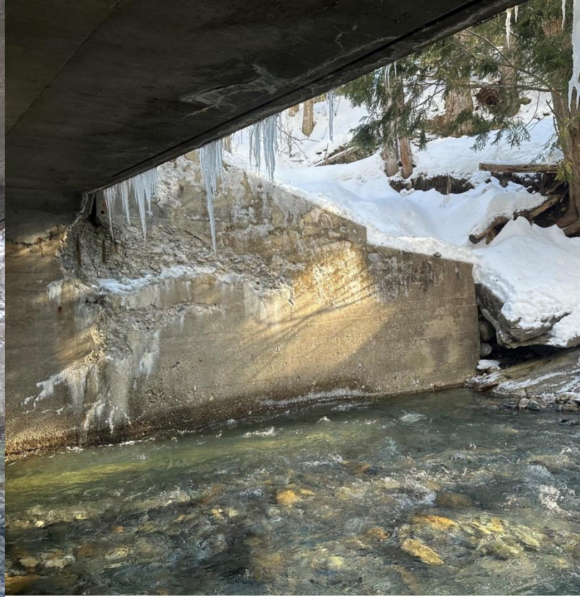
Abutment 2 Downstream Wingwall
