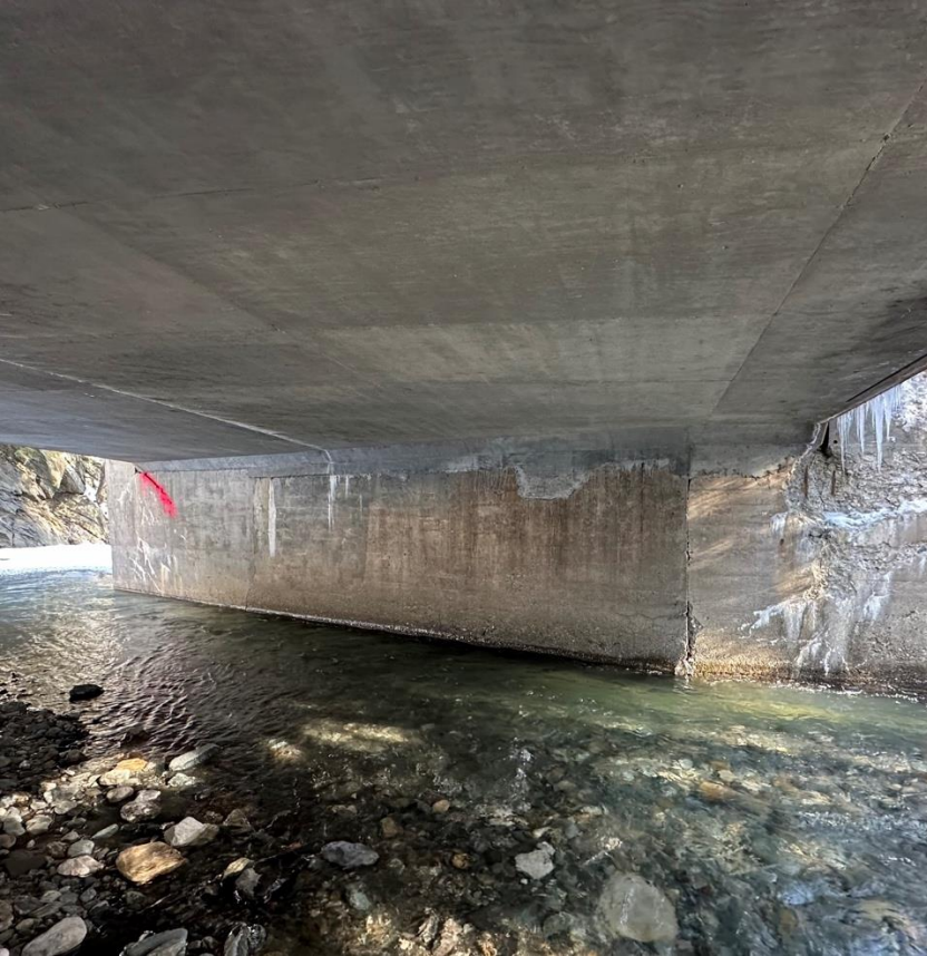
Underside of Deck
