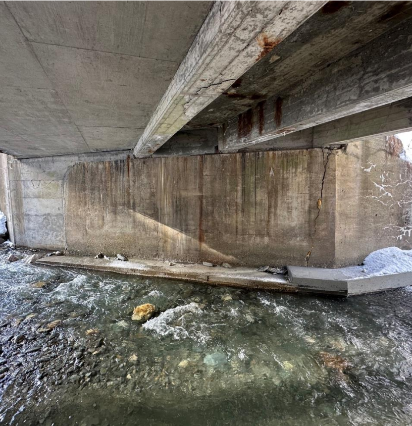
Underside of Deck
