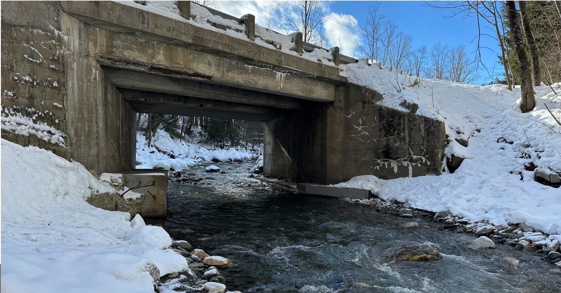
Plymouth ER P23-1(328) VT Route 100A– Bridge #7 over Pinney Hollow Brook
